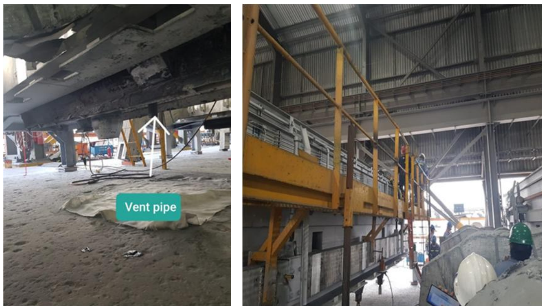
Figure 4. Left: vent pipe; Right: ventilation installation in the pot repair.
