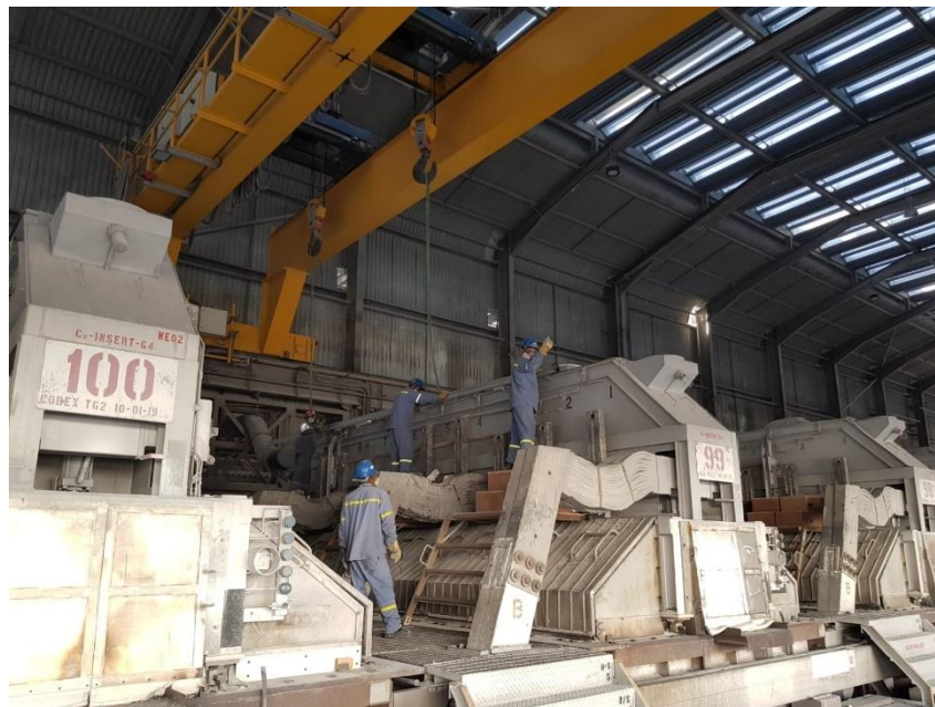
Figure 7. Lifting using the construction crane.
